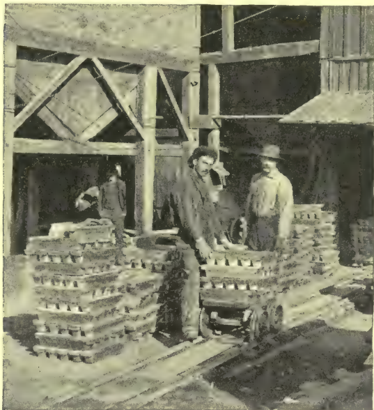
BULLION AT THE AMERICAN SMELTER, LEADVILLE, COLORADO
